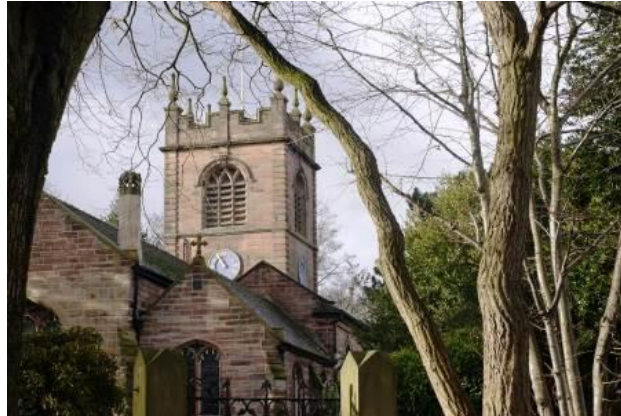
Views of the church from the west along Church Road
