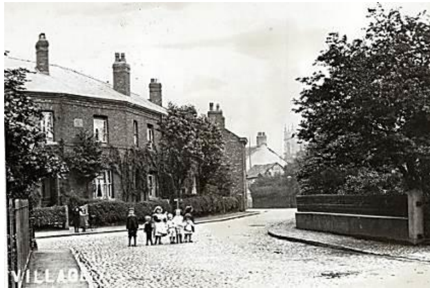
View along Church Road towards the church in 1906
