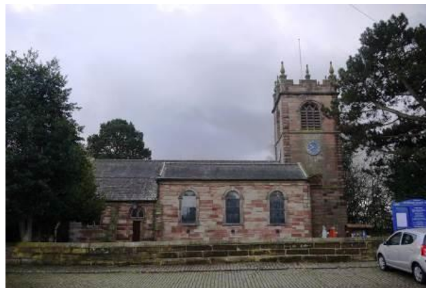
View of the north elevation of the church, from Church Road
