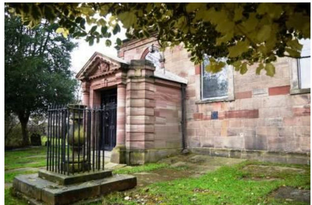
The south elevation of the church, showing the 1909 porch and the listed sundial
